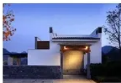
Household Energy Storage
