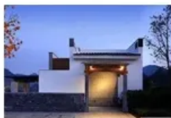
Household Energy Storage
