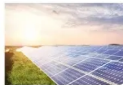
Energy Storage System
